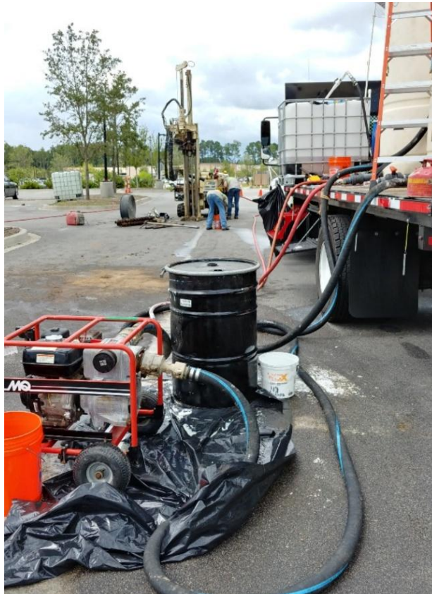
Figure 5. Mixing and injection equipment at the site.
