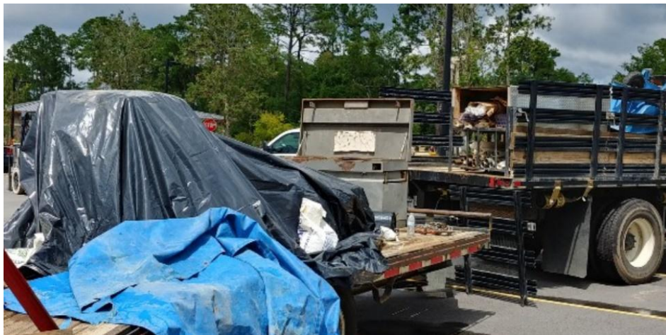
Figure 2b. Amendment materials and equipment staged for injection.
