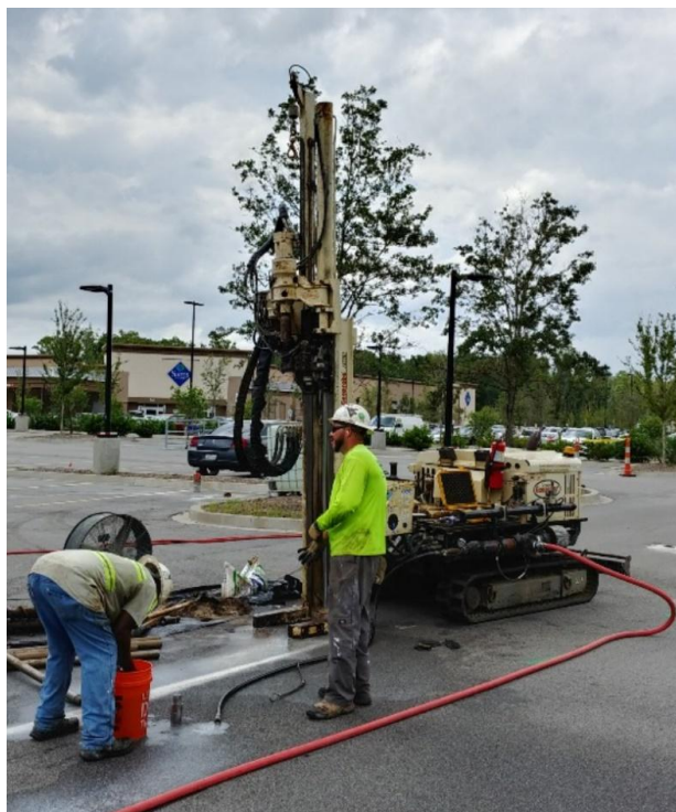
Figure 6. Injection activities at the treatment site.
