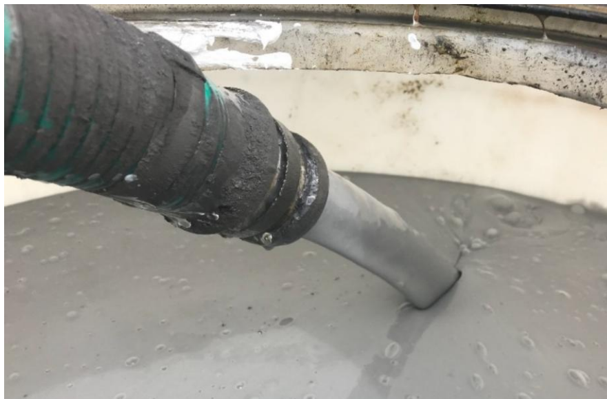
Figure 4. Prepared amendment slurry during field mixing.
